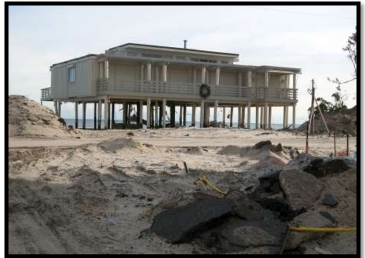
Residential home being raised to adhere to Base Flood Elevations. Photo courtesy of FEMA
