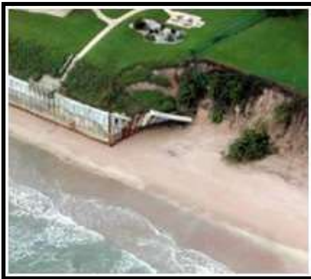
The effect of a bulkhead on adjacent property. Photo: US Fish and Wildlife Service.
