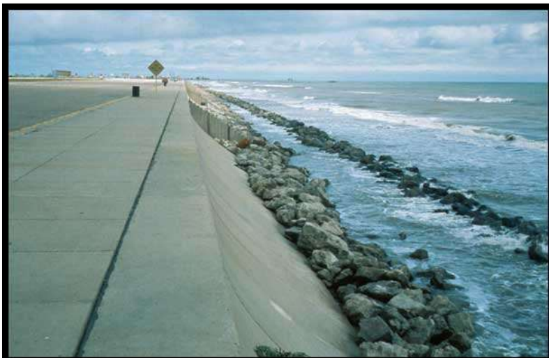
Hard structures, such as the Galveston seawall, can increase erosion of adjacent beaches. Source: USGS.
