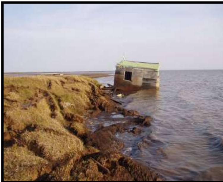
A CABIN ALONG ALASKA'S ARCTIC COAST WASHED INTO THE OCEAN BECAUSE THE BLUFF BENEATH IT ERODED AWAY. PHOTO: BENJAMIN JONES, USGS.
