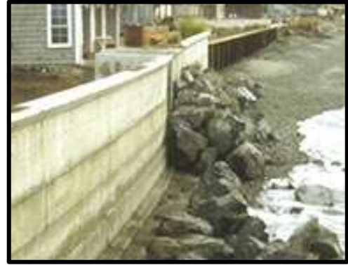
Narrowed beach in front of a bulkhead. Photo: WA Department of Ecology.
