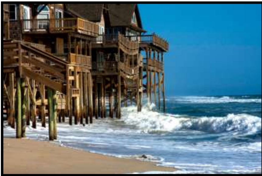
Rodanthe, North Carolina, September 2, 2011. These raised homes once had yards of beach between them and the sea, until Hurricane Irene hit the coast. Photo: FEMA / Tim Burkit.
