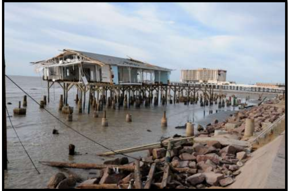
Storm surge damage from Hurricane Ike in Galveston, TX (2008). There were once 4 piered structures along this section of the seawall. Photo: NOAA Flower Garden National Marine Sanctuary.
