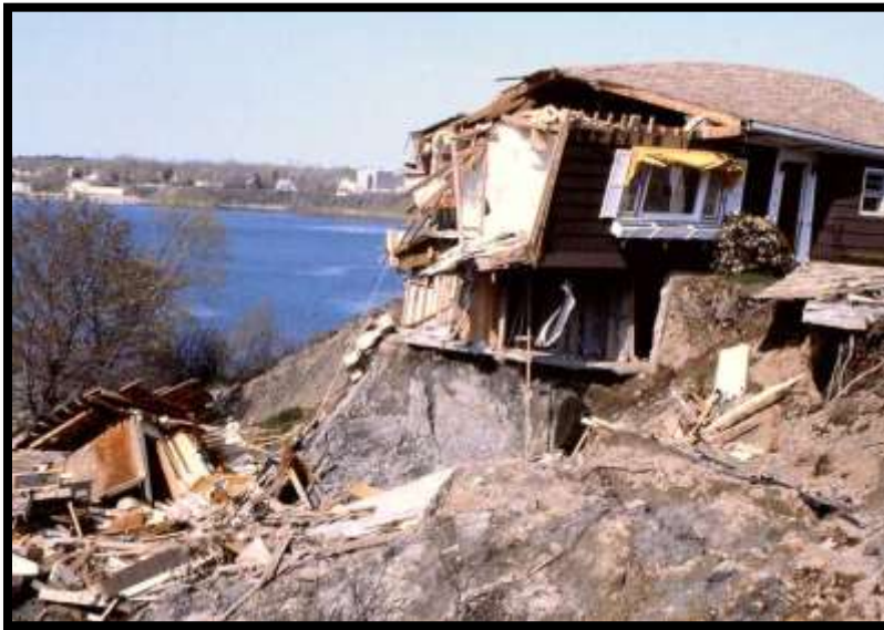
A clay bluff on the north shore of Rockland Harbor failed in 1996. This landslide formed a new scarp about 200 feet landward of the original top of the bluff in just a few hours. Two homes were destroyed. Photo: Maine Department of Agriculture, Conservation, and Forestry.
